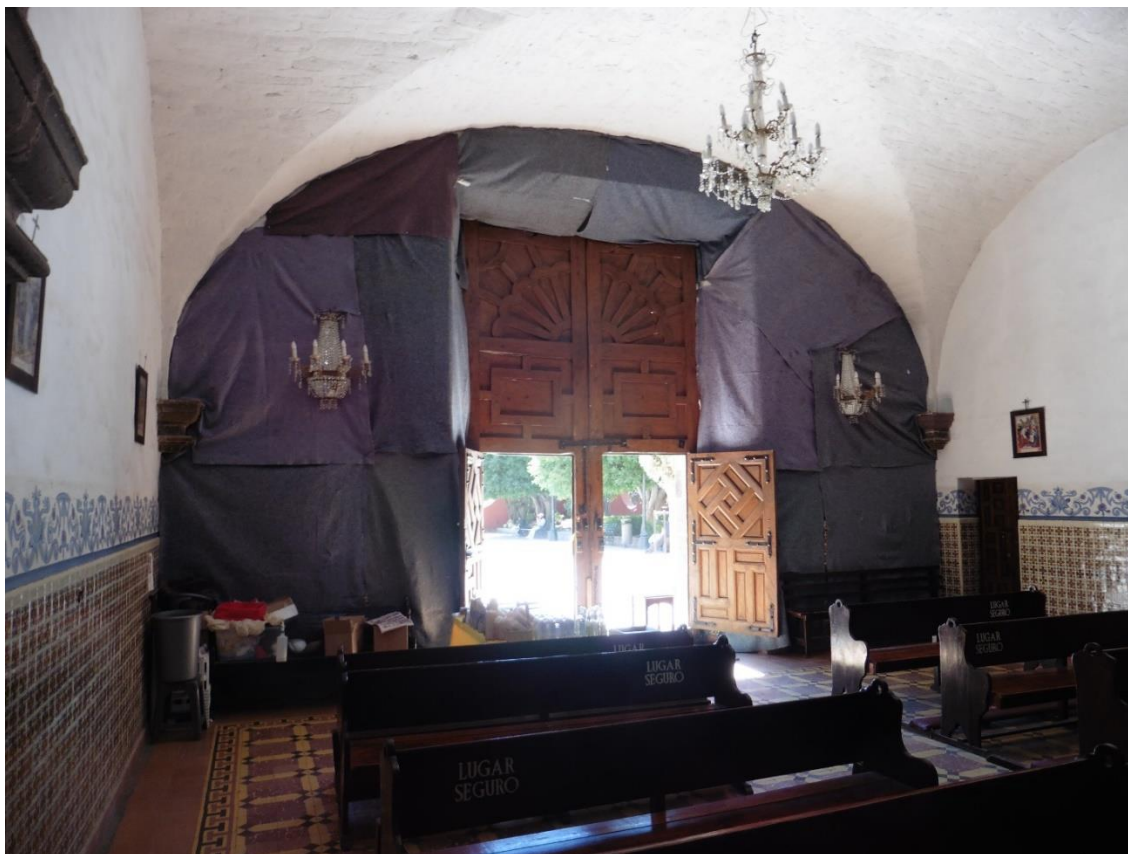
Figure 17 Moving Blankets Attached to Rear Wall to Absorb Reflections
